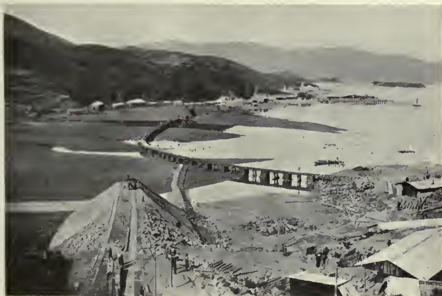
CONSTRUCTION SCENE ON THE KOWLOON-CANTON RAILWAY.
