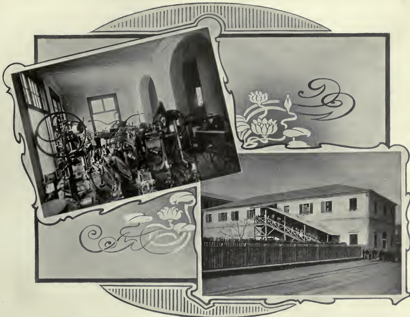
GODOWNS AND MACHINERY SHOWROOMS OF SIEMSEN & CO. AT HANKOW.
