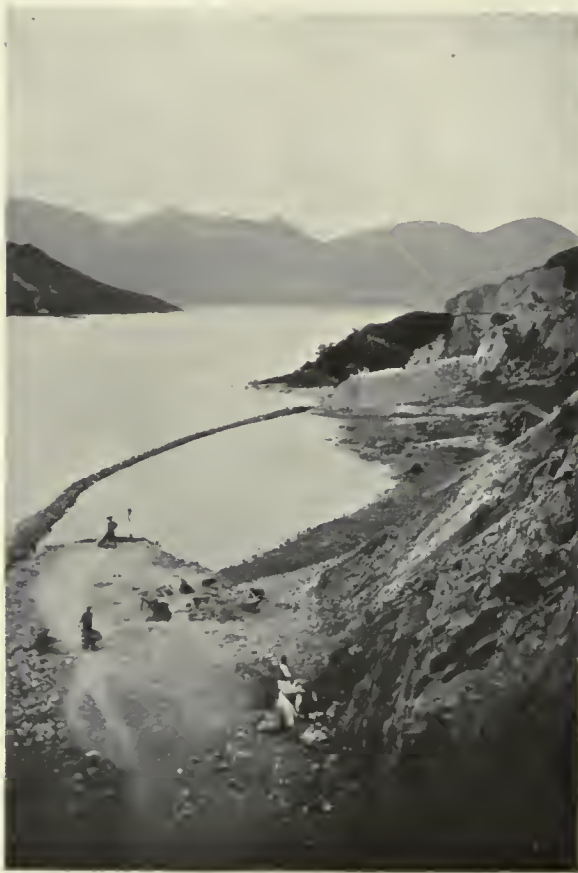
CONSTRUCTION SCENE ON THE KOWLOON-CANTON RAILWAY.
