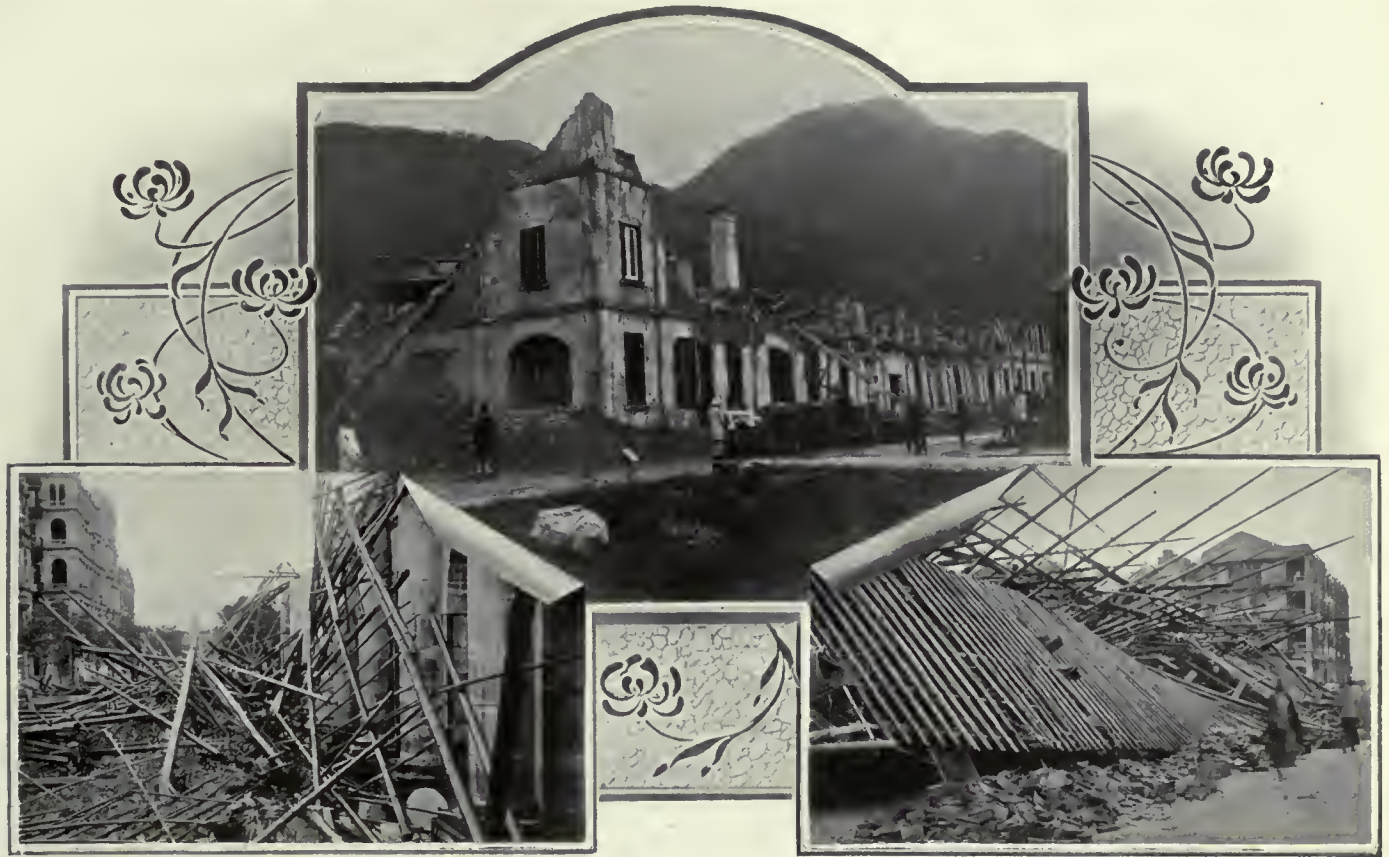
THE GREAT TYPHOON—DAMAGE DONE ON SHORE.
