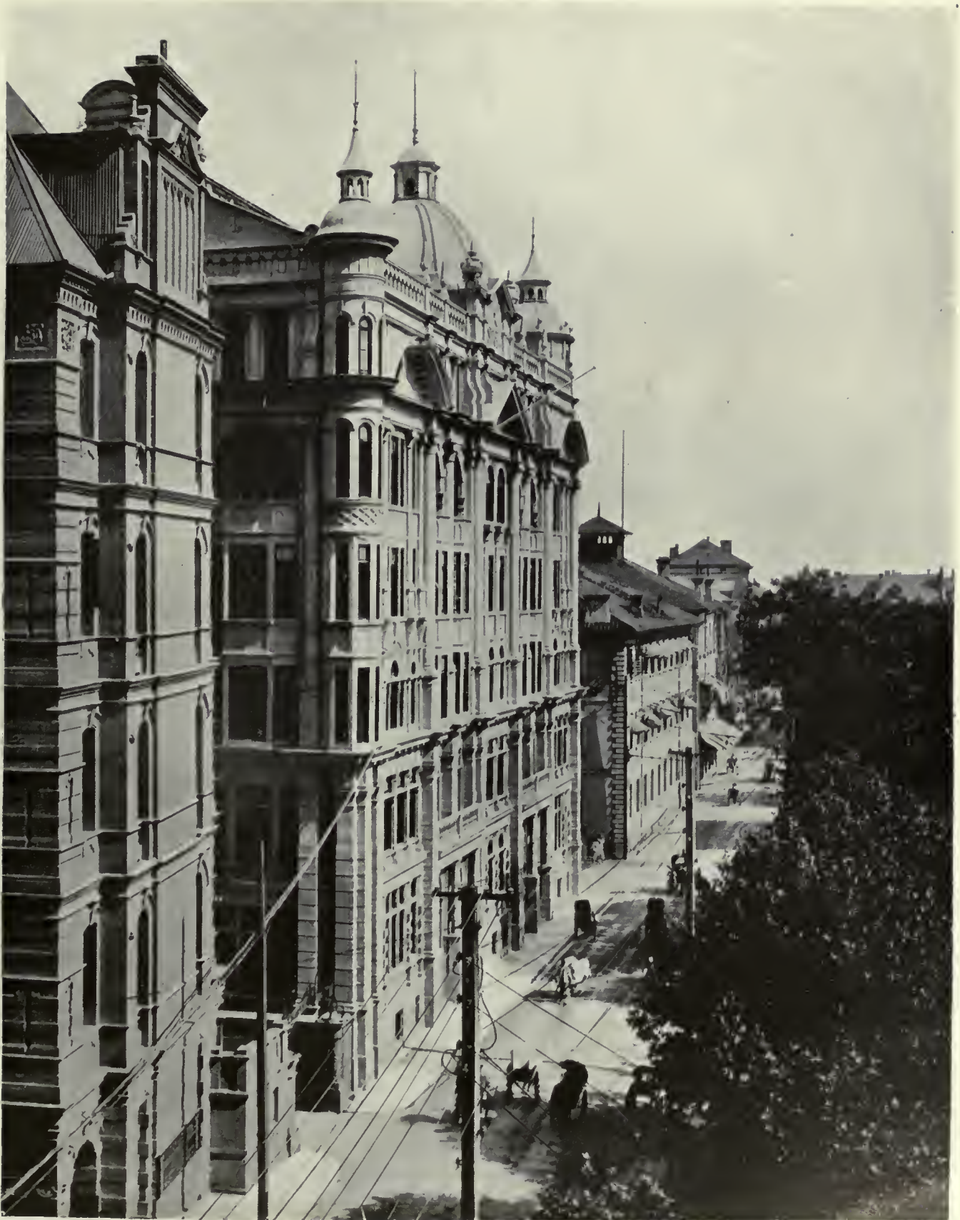
THE SHANGHAI MUTUAL TELEPHONE COMPANY'S NEW PREMISES IN KIANGSE ROAD.
