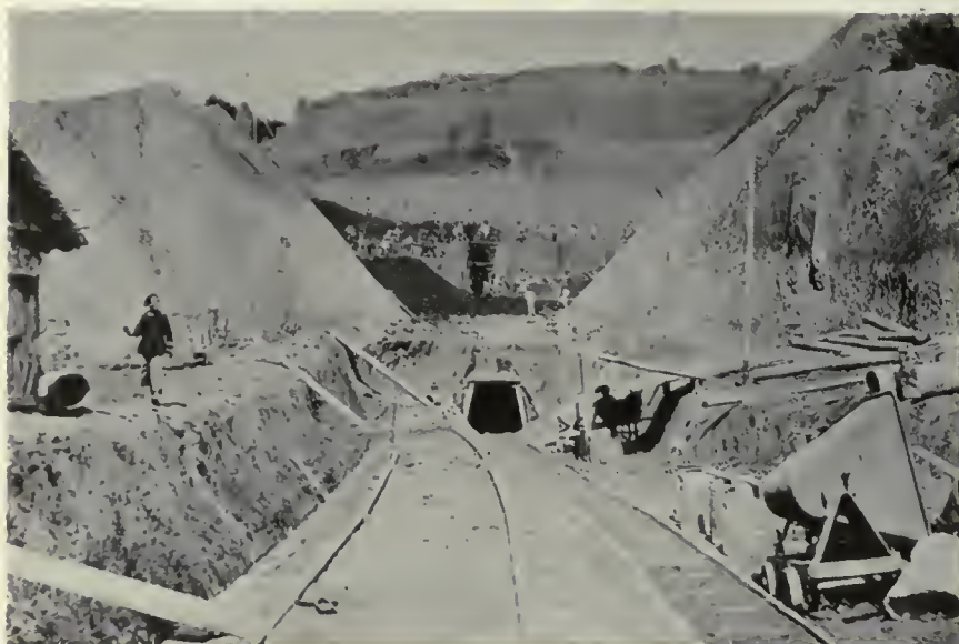
CONSTRUCTION WORK ON THE CHINKIANG TUNNEL— SHANGHAI-NANKING RAILWAY.
