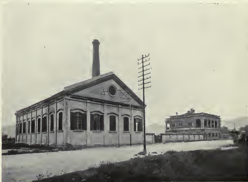
CHINA LIGHT AND POWER COMPANY, LTD.—GENERAL VIEW OF WORKS AT KOWLOON.
