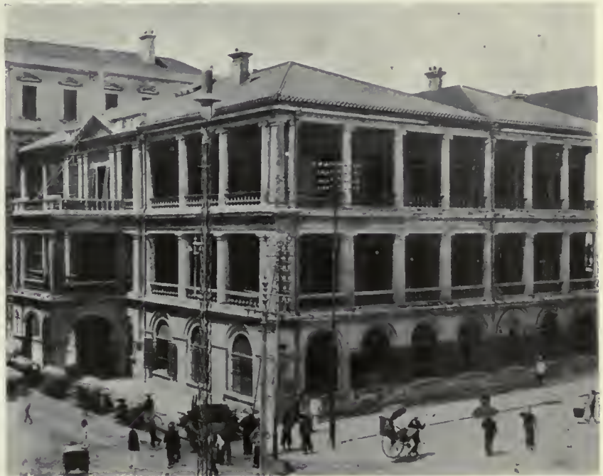
JARDINE, MATHESON & CO.'S OLD PREMISES. (Demolished October, 1907.)
