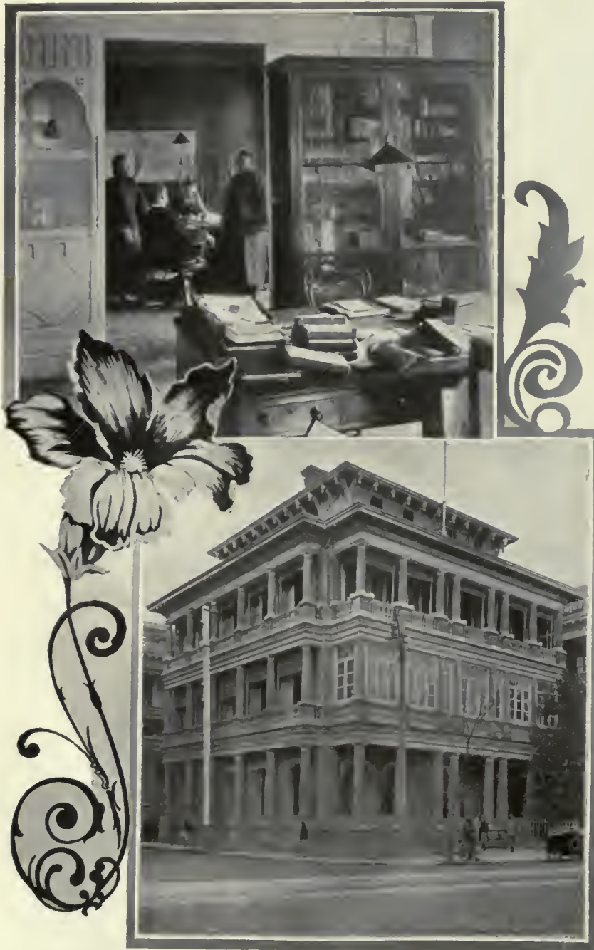
THE PREMISES OF TELGE & SCHROETER, ON THE BUND.
