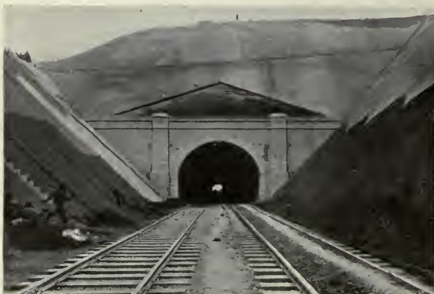
THE CHINKIANG TUNNEL—SHANGHAI-NANKING RAILWAY.
