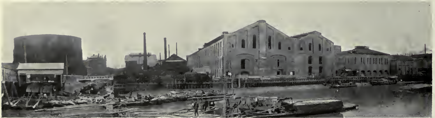
THE GAS WORKS.
