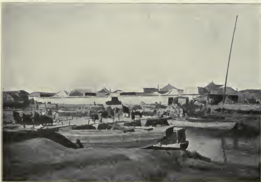
A PONTOON BRIDGE, TIENTSIN.
