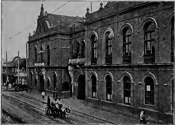
TOWN HALL, NANKING ROAD
