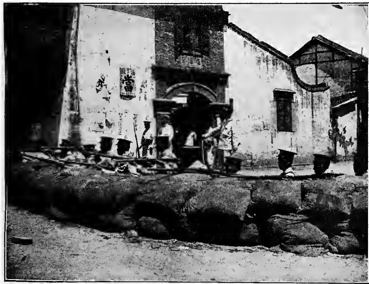
Northern entrenchment close to the Arsenal Gate, opposite Pont St. Cathérine.
