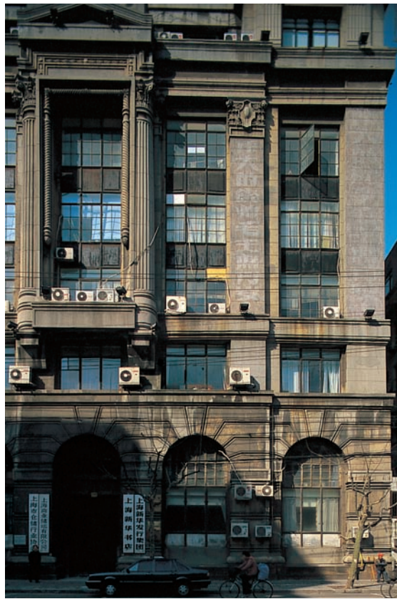
Left The facade of one of Shanghai's offices in the former Central District with the faded slogan 'Long Life Great Leader Chairman Mao' painted on the central pilaster
