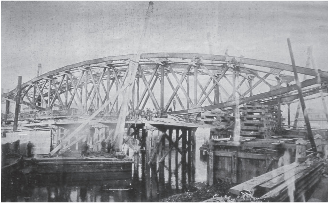
Left The Zhejiang Road Bridge under construction, 1908
