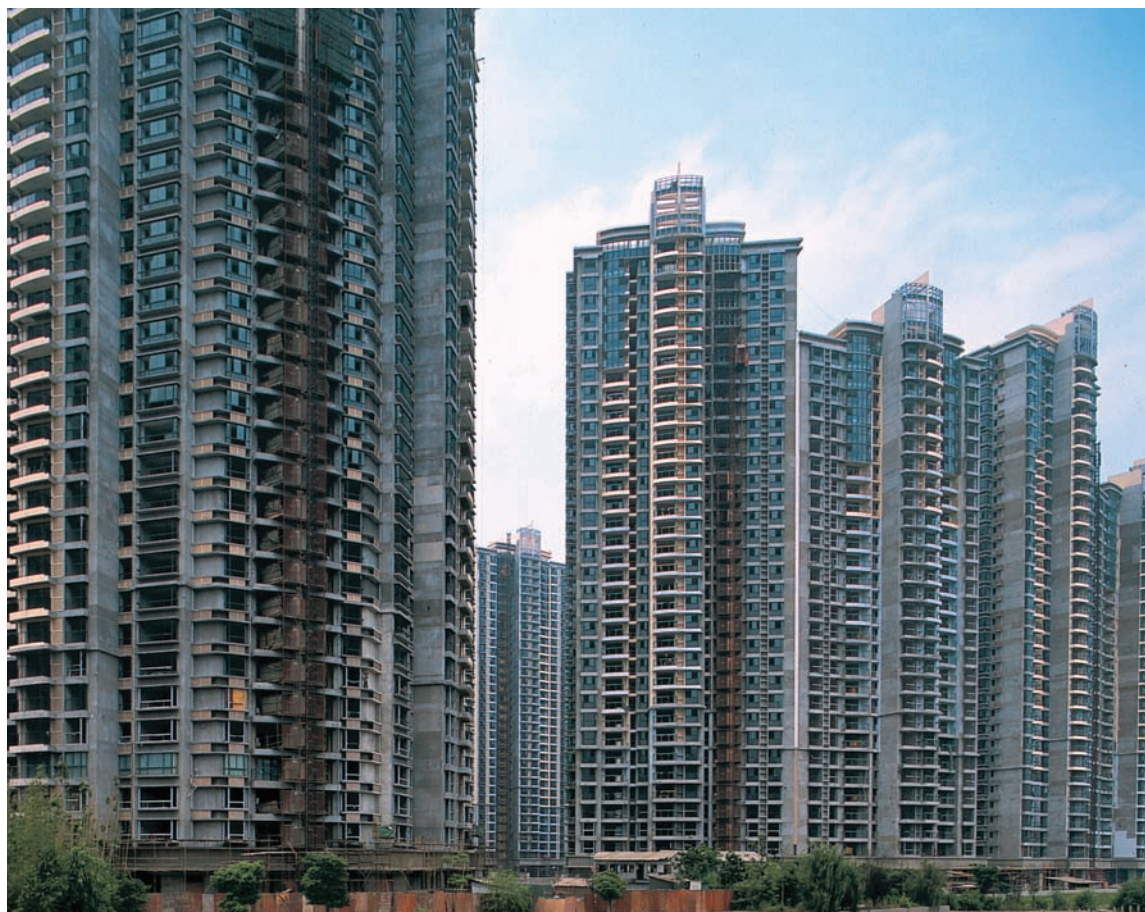
Left New residential towers being built north of Suzhou Creek
