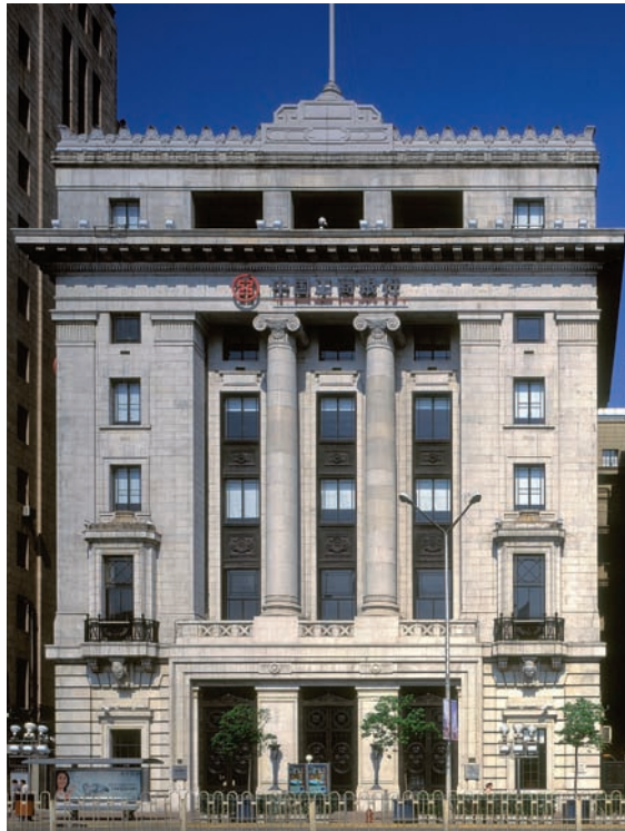
Right and far right The former Yokohama Specie Bank
