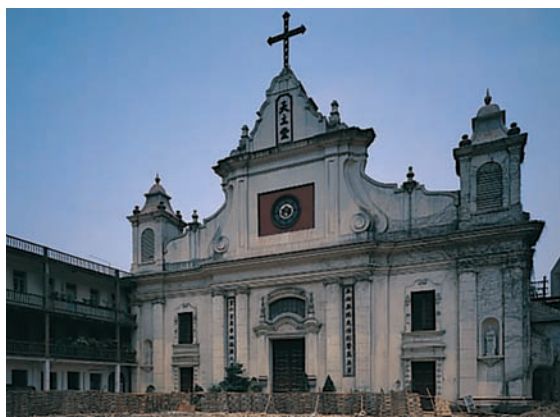
Left The exterior of Dong Jia Du Cathedral being restored in 2005 and below its interior
