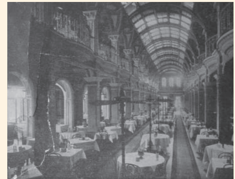
Above The barrel-vaulted glass roof of the dining hall
